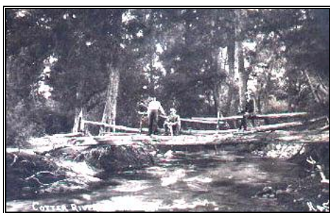
Above: An early photograph with title of First Bridge across the Cotter River. Loaned by Alison Neiberding.
