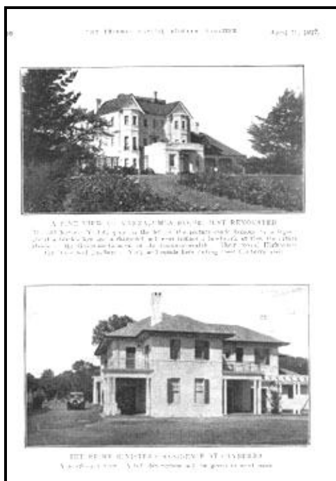
Top photograph – Yarralumla House 1927 and below The Prime Minister's Lodge. Photograph in The Federal Capital Pioneer 1927.
